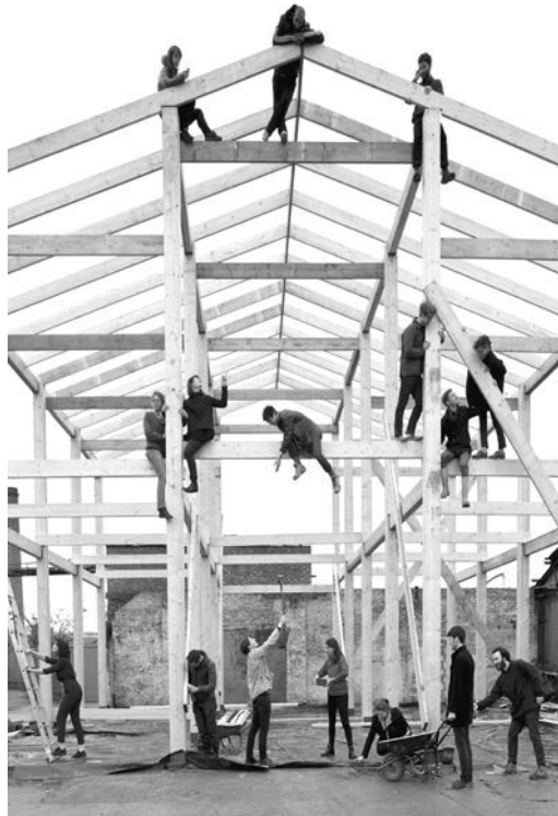
Figure 22 Assemble collective's Yardhouse studios for London creatives under construction (Courtesy Assemble)
